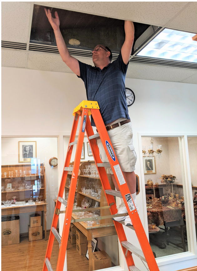
David Ray went up the ladder to change a few ceiling tiles. Thank you!
