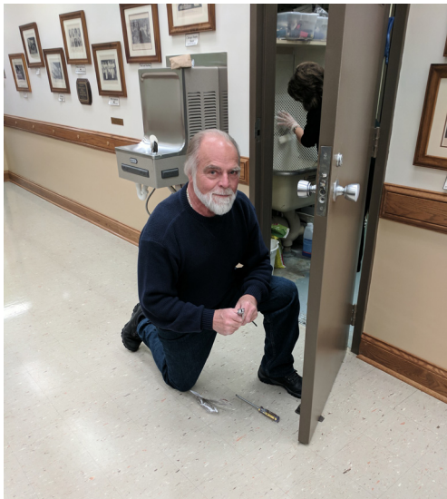
Roger Loucks helped out by replacing a door holder.
