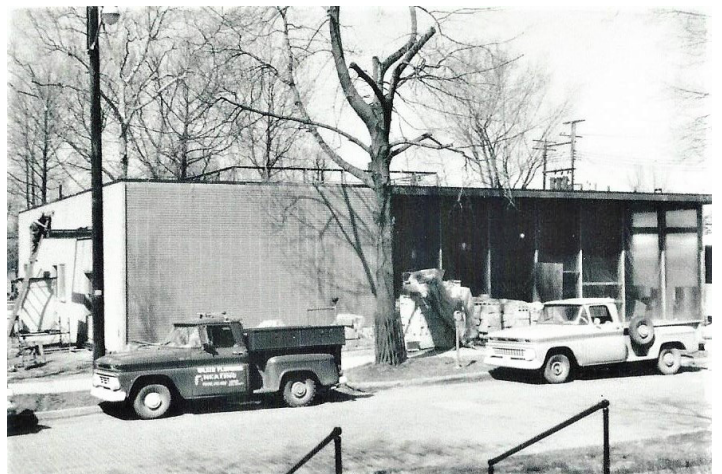
Ohio Power Building Construction
