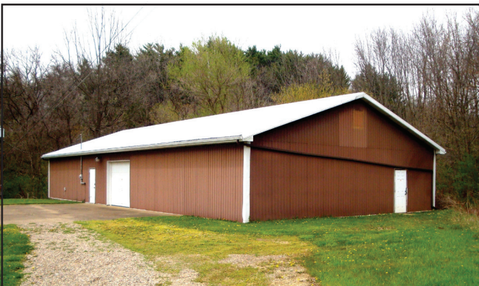
The NCC Mould Storage Building looks fresh and clean after the metal roof was painted.
